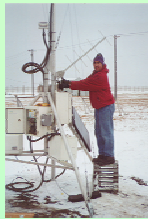
Wily Splain helps install a NEWNET station in Barrow.
