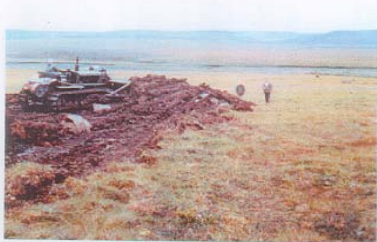
Figure 1-4: Bulldozer Covering the Radioactive Tracer Material at the Chariot Site – 1962.
